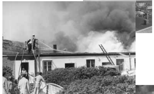
Baracke Am Sandwall 1973
